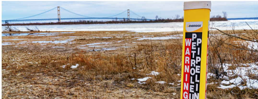
RIGHT: An Enbridge Energy “Warning: Petroleum Pipeline” at the site of the Line 5 oil pipeline site at the Straits of Mackinac between Lake Michigan and Lake Huron. Photo Credit: Tony Webber
