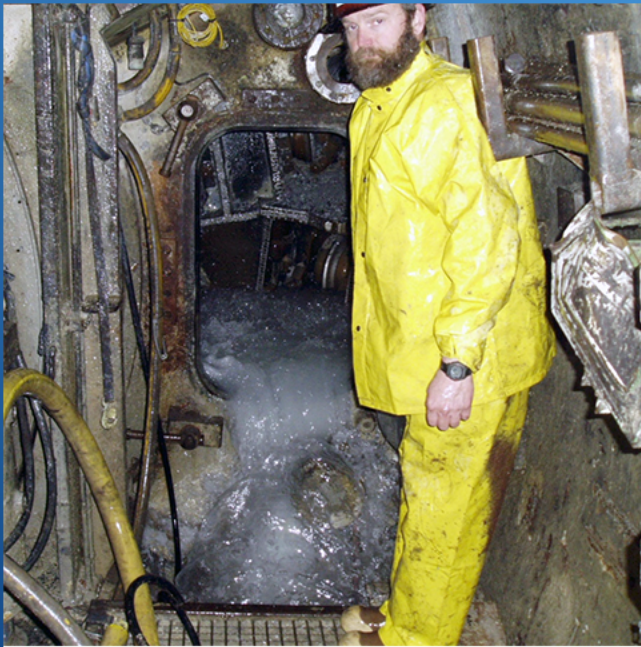
PHOTO: Water discharge through a shielded Tunnel Boring Machine's open pressure bulkhead, preventing maintenance and repair work. McMillen Jacobs Associates for the State of Michigan 11 .
