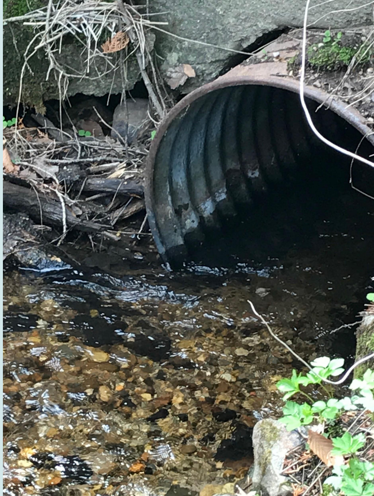
Culvert used to document the historical high water mark
